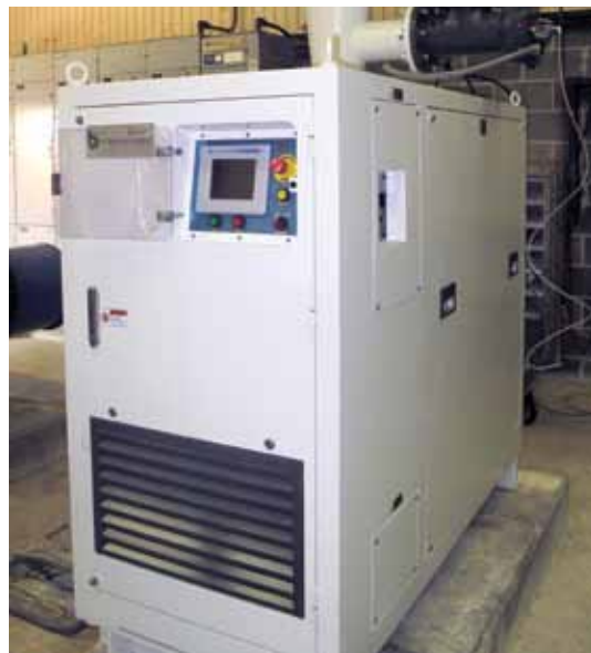
Unit 3 in the blower room at Longview’s Grace Creek Wastewater Treatment Plant is a new APG-Neuros NX 150 aerator blower that can be used to supply air to any of the four aeration basins at the facility.
